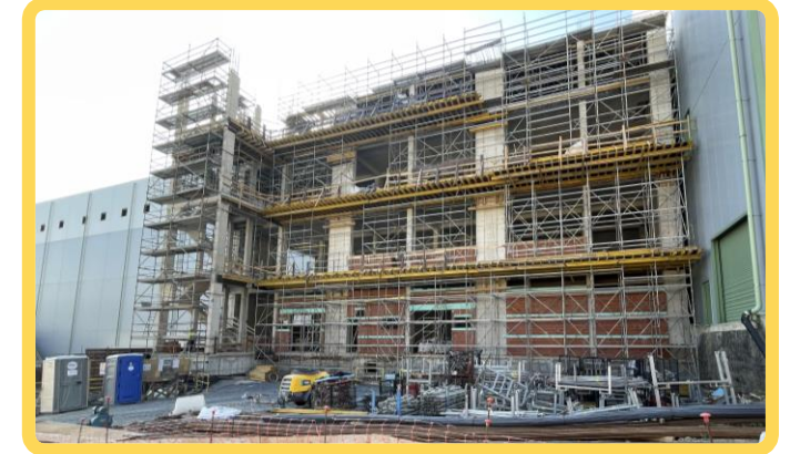
Process control building
